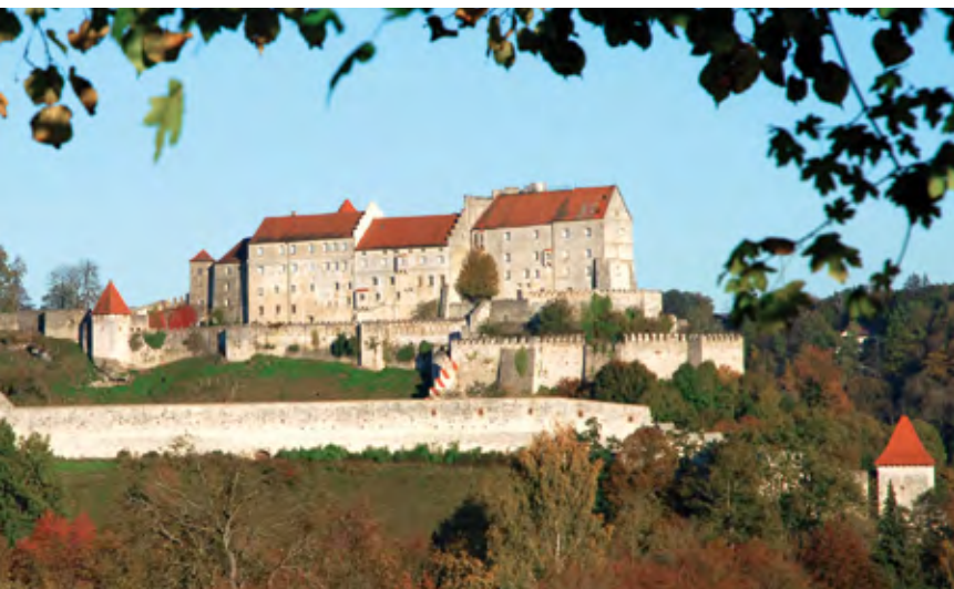
Historic building: view of the main castle
